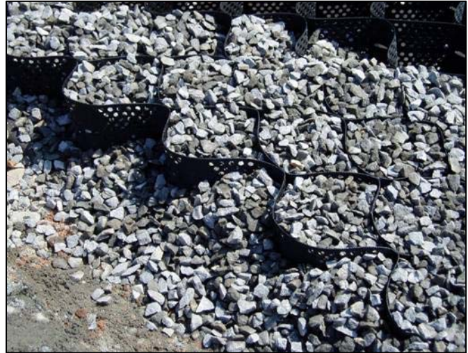
One type of porous paving system (shown above) involves filling a synthetic grid with clean gravel.
