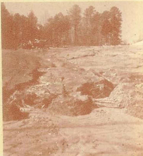
Erosion from unprotected construction sites harm our rivers, lakes, and streams.
